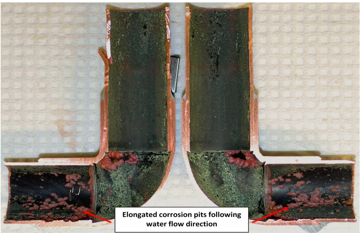
Figure 4.9 Photograph showing erosion corrosion (elongated corrosion pits following water flow direction) in a copper domestic water line.
