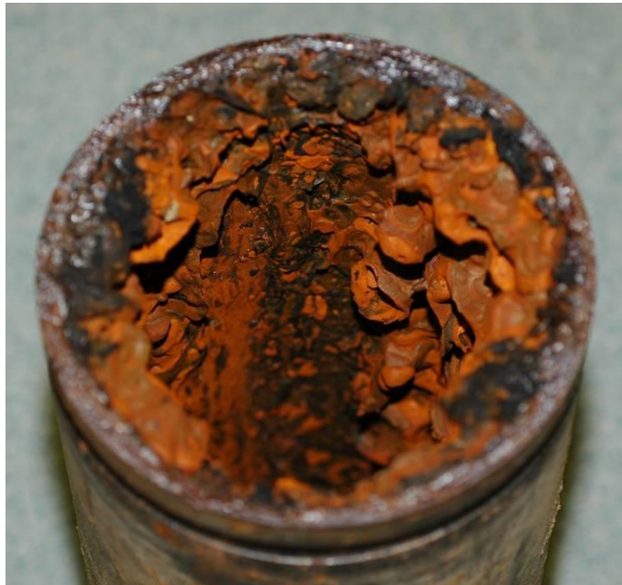
Figure 4.15 Photograph showing a corroded/leaked steel sprinkler pipe (4 inch dia.) with many tubercles. MIC caused by SRB was identified to be a likely contributing factor to pipe corrosion.
