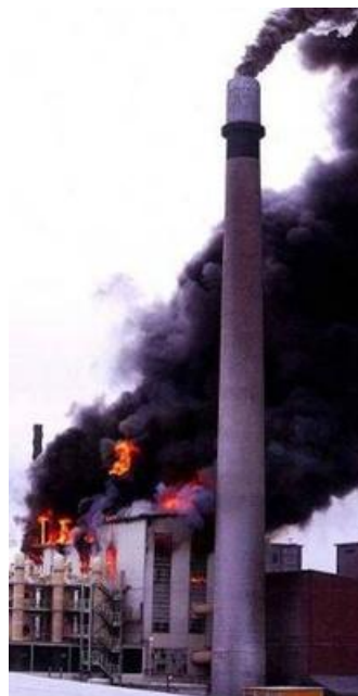
Figure 6.4 Photographs of fire incidents. (A) An unsprinklered steel pickling facility with plastic ductwork system, and (B) An unsprinklered facility with corrosive environment.
