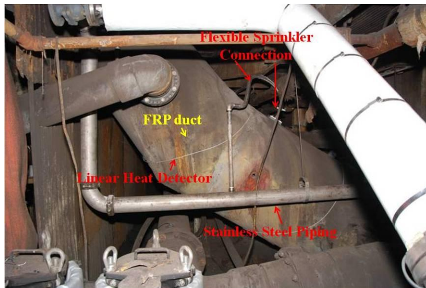
Figure 6.5 Representative photograph showing part of the fire protection system protecting the main FRP exhaust duct.
