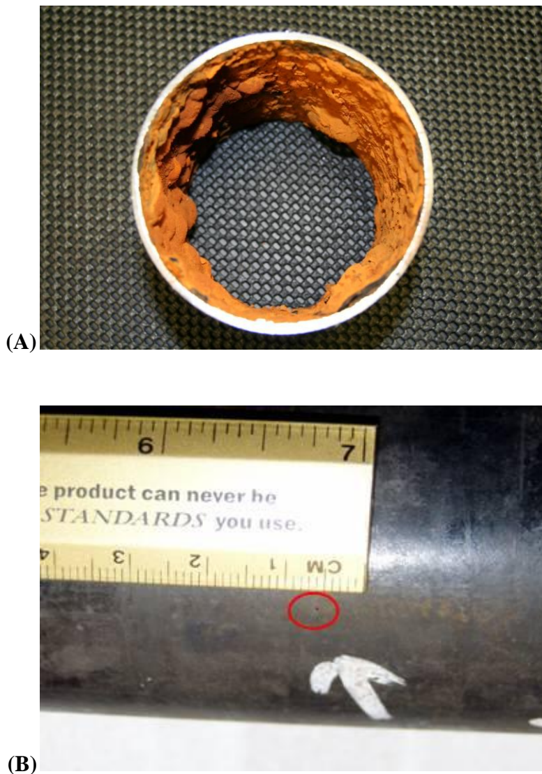
Figure 4.16 Photograph showing tubercles and pinhole (circled) leakage of steel sprinkler pipe in wet pipe systems. (A) Tubercles heavily formed inside a steel sprinkler pipe (4 inch dia.). (B) Pinhole (circled) leakage on a steel sprinkler pipe.
