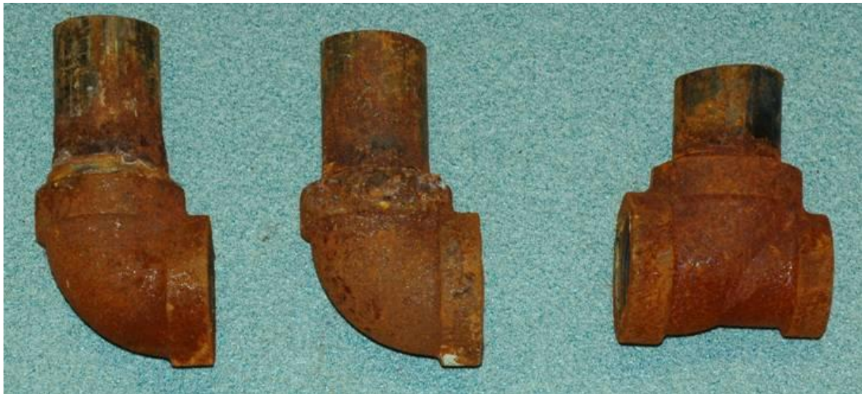
Figure 4.2 Uniform corrosion of steel sprinkler pipe joints (2 inch dia.) in a wet pipe system caused by water leakage past their thread joints.
