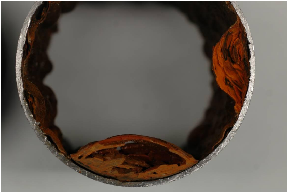
Figure 4.19 Photograph showing the cross section of non-MIC tubercles in a NPS 4 Schedule 10 steel sprinkler pipe. Irregular shapes of cavities are visible inside two larger tubercles.
