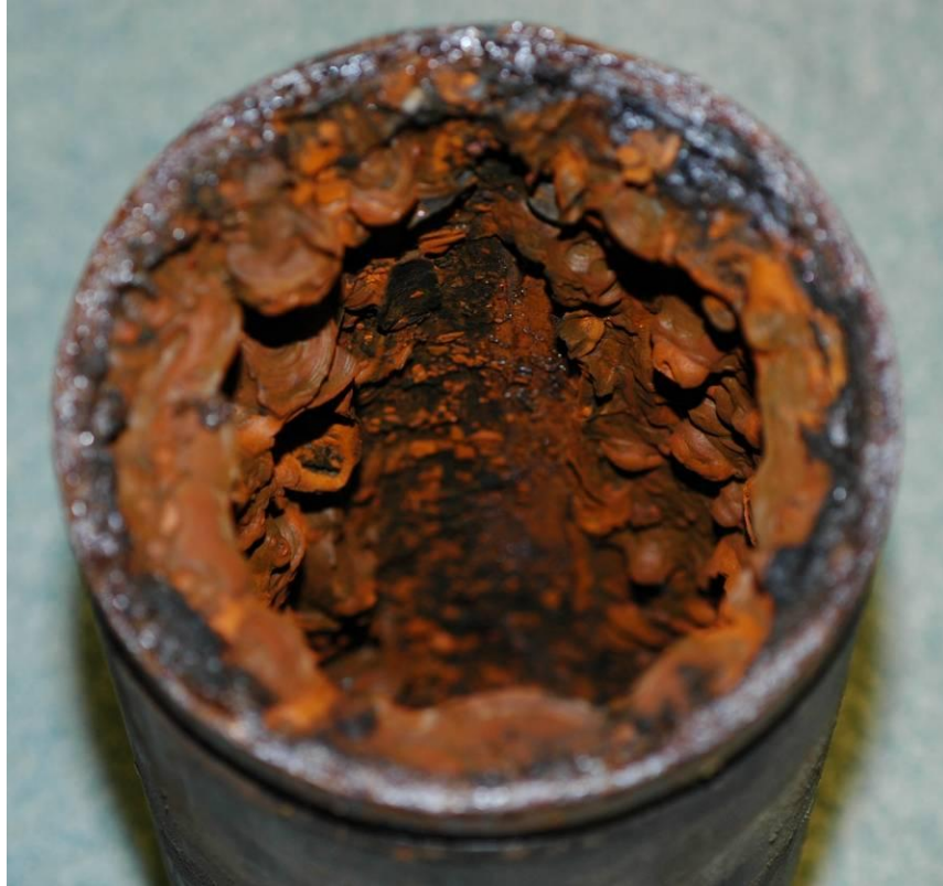
Figure 5.10 Photograph showing extensive tuberculation and deposit buildup for a portion of the Pipe Sample #1 in Table 5.2.
