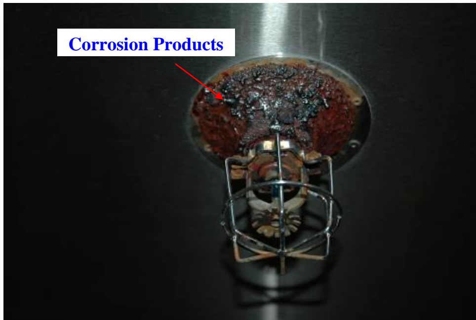
Figure 4.3 Photograph showing galvanic corrosion damage of a less noble steel connection (anode) contacting a large noble stainless steel plate (cathode) inside a high humidity environmental chamber.
