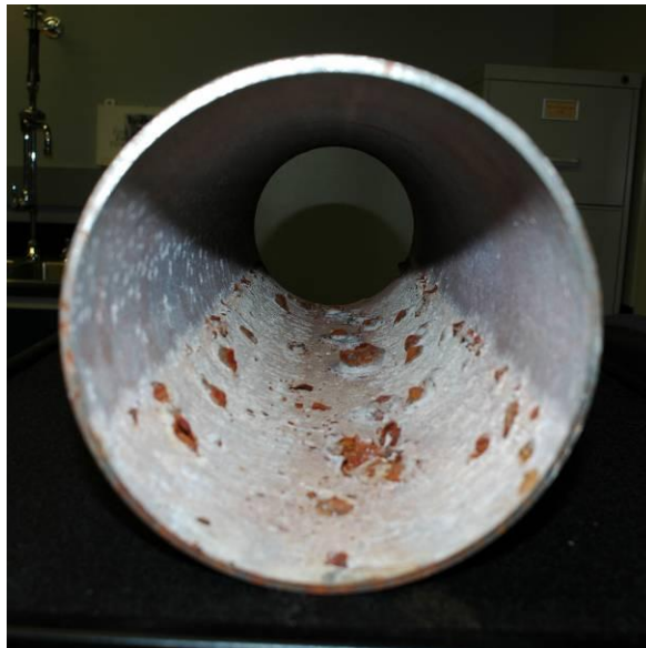
Figure 5.7 Photograph showing corrosion of galvanized steel pipe (NPS 6, Schedule 10) where residual water filled about 40% of the pipe's volume in a dry pipe system.
