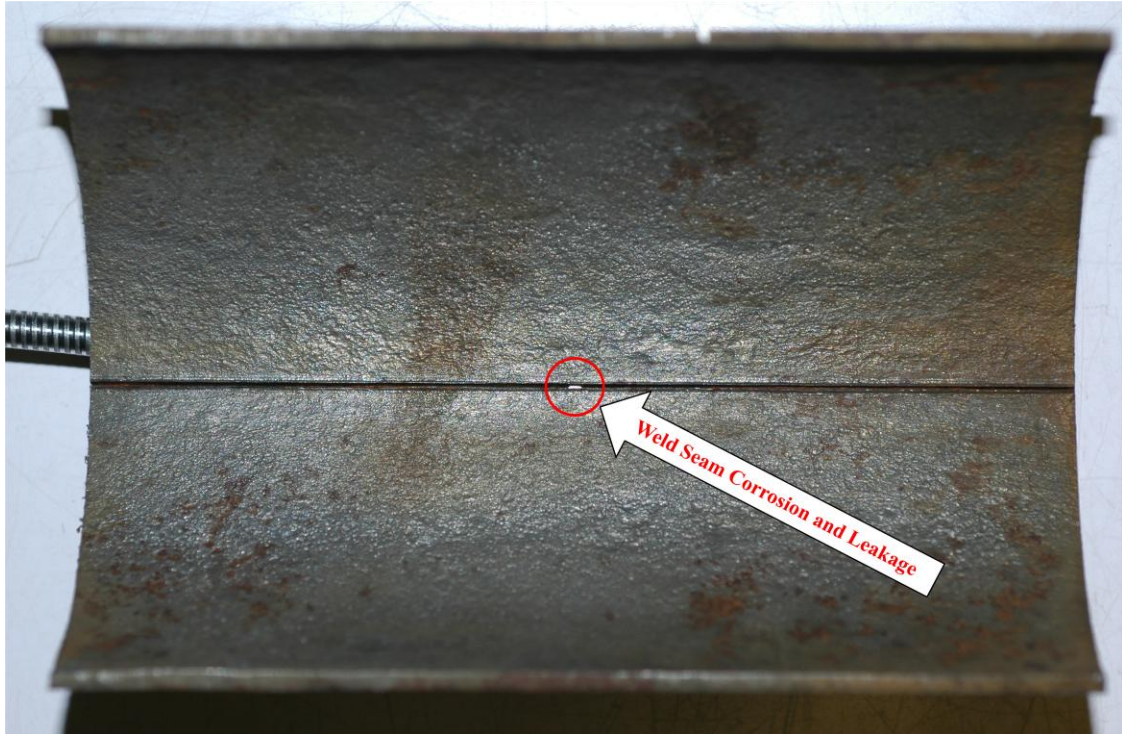
Figure 5.2 Photograph showing preferential grooving corrosion on pipe weld seam with a 1 mm pinhole leak in a wet pipe system, after removing corrosion products inside an NPS 3 pipe.
