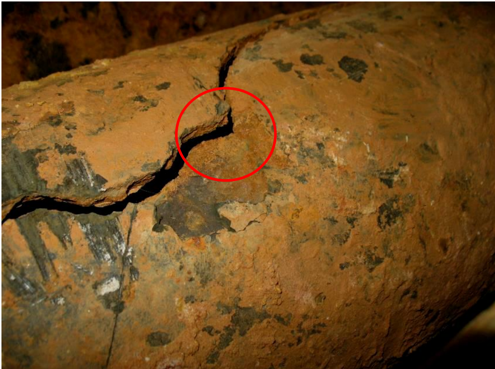
Figure 4.7 Photograph showing a ruptured underground water main (8 inch dia.) with circled area indicative of graphitic corrosion.
