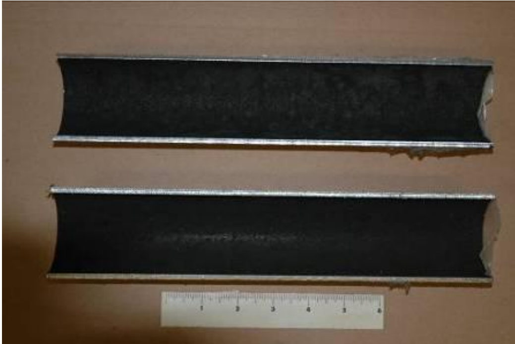
Figure 4.20 Photograph showing steel pipe in a wet pipe system with limited corrosion after forming a layer of black magnetite and depleting oxygen inside this piping system.
