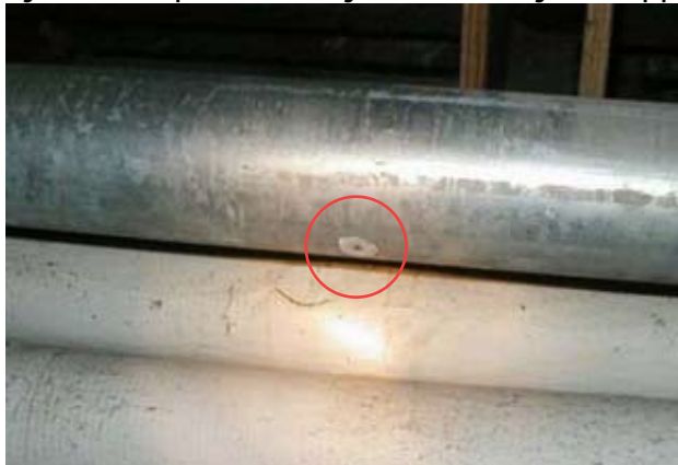
Figure 3 Pinhole perforation through 3-inch-diameter galvanized pipe
