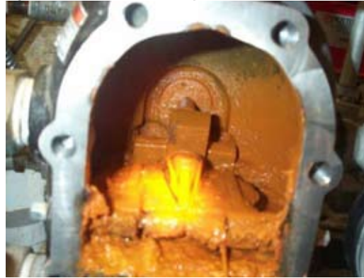
Figure 4 Interior condition of preaction valve
