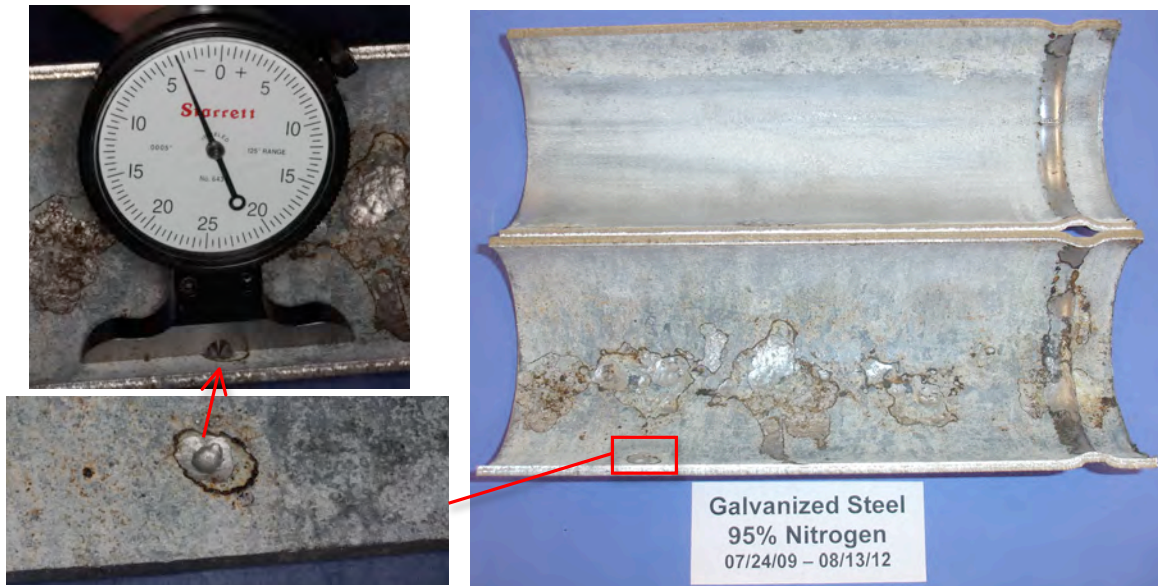
Figure 6. Galvanized piping after 1116 days exposure while approximately half-filled with water and under 95% nitrogen supervision. Note localized pitting at locations where zinc coating has been breached.
