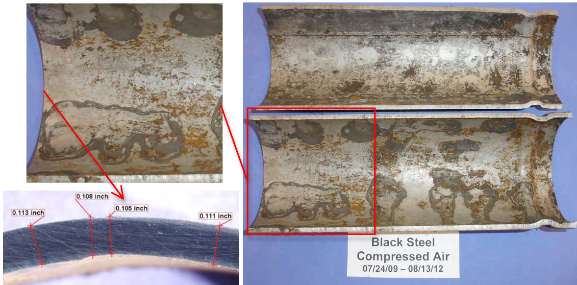
Figure 2. Composite image of black steel piping after 1116 days exposure while approximately half-filled with water and under compressed air supervision. Note uniform thinning of pipe wall and absence of any localized pits.
